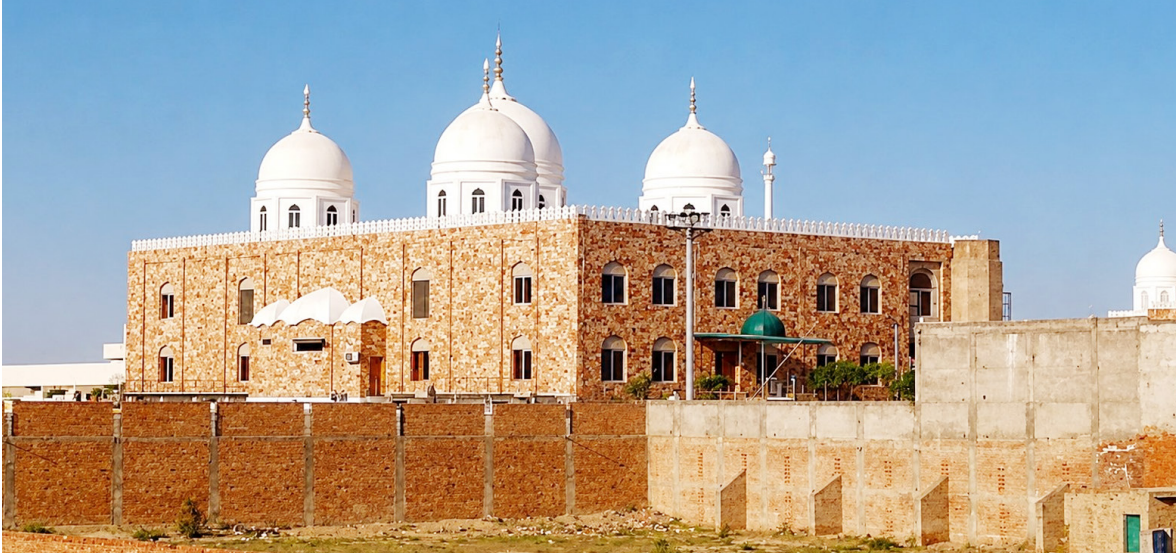
The newly rebuilt Markaz Subhanallah complex in Bahawalpur, Pakistan, reportedly reconstructed after sustaining extensive damage during India’s Operation Sindoor strikes in May 2025.
