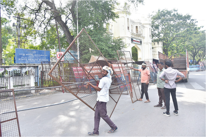
Workers installing barricades near Secratariat ahead of Monsoon Assembly session in Hyderabad on Saturday. Munsif Bureau
