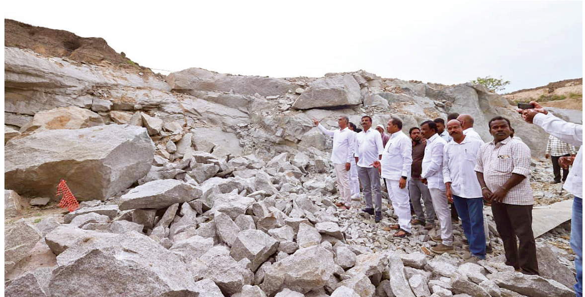
BRS deputy floor leader in assembly T. Harish Rao has warned that rock blasting near Mallannasagar reservoir could pose a threat to the dam and demanded an immediate halt to the work. Inspecting the reservoir with BRS leaders on Thursday, Rao alleged that blasting had been carried out for two months about 200 metres away from the reservoir without necessary permissions.
